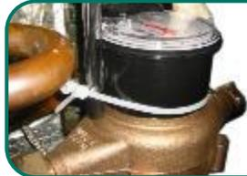
Read out water usage data from a sensing device isolated from the main unit
